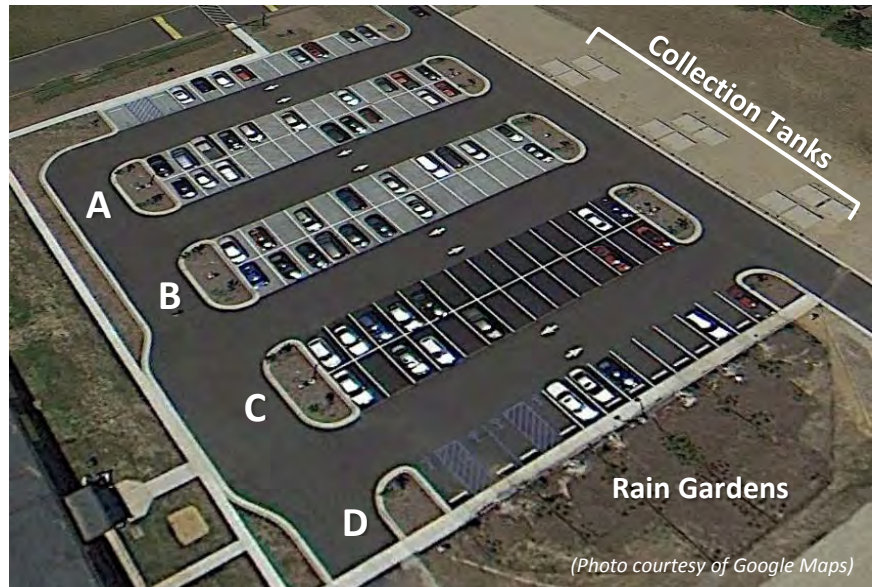
Figure 1. Aerial view of EPA's Edison Environmental Center permeable parking lot: (A) permeable interlocking concrete pavers, (B) pervious concrete, (C) porous asphalt, (D) conventional asphalt.
