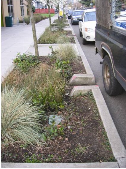
Curb cuts allow water to flow into a bioretention area
