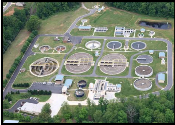
Below: City's New 8 MGD Advanced Water Reclamation Facility
