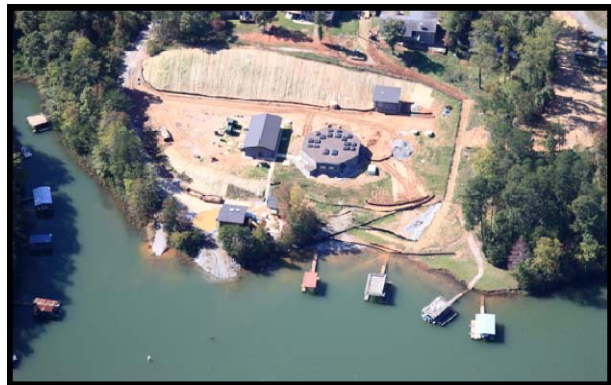
Below: City's New 105 Million Gallon Per Day Raw Water Inake Facility
